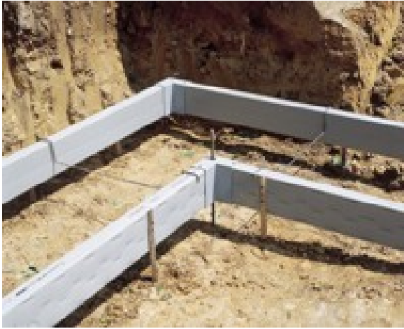
Figure 2. Form-A-Drain corner assembly
