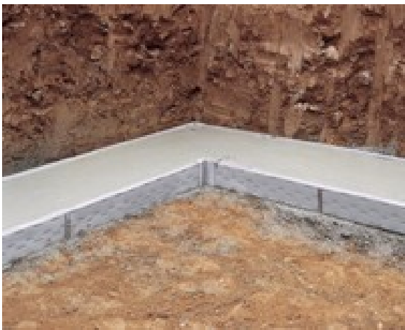
Figure 3. Form-A-Drain corner assembly after concrete placement
